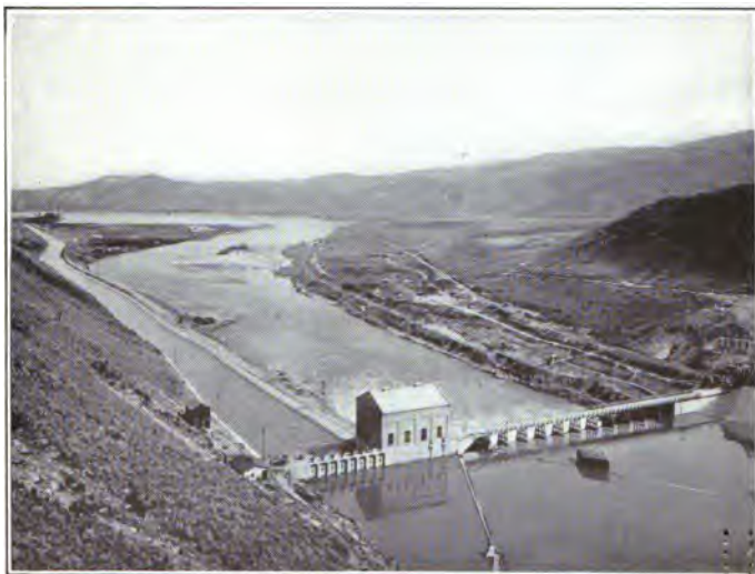
RECENT CONCRETE DAM, BOISE RIVER, IDAHO. Power plant and head of main canal, typical gravity diversion from river.
